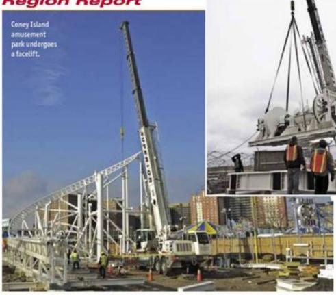
The Terex T-550-1 truck crane's 110-foot main boom and 50-ton capacity proved to be a great asset in positioning the Steeplechase rollercoaster's 18.6-ton motor in place.
